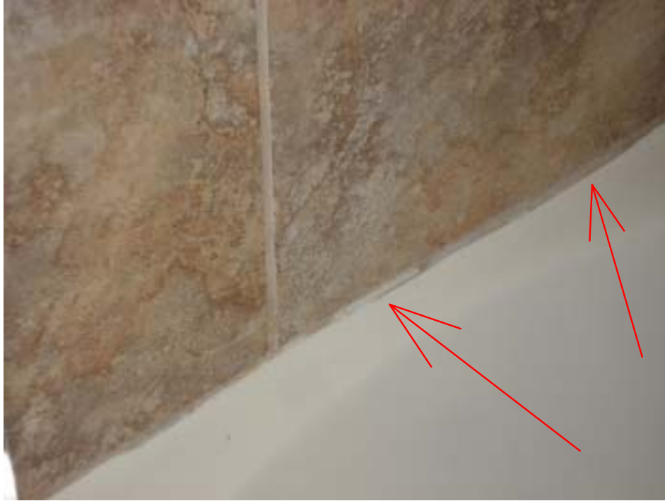
PIC 7: Grout repairs for East 2nd level bathroom room.
