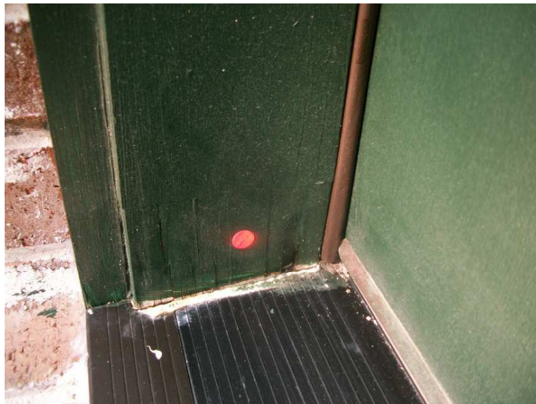
Door casing at the second floor entry door.
