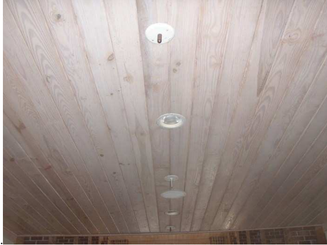
Fly Spray System At The Ceiling
