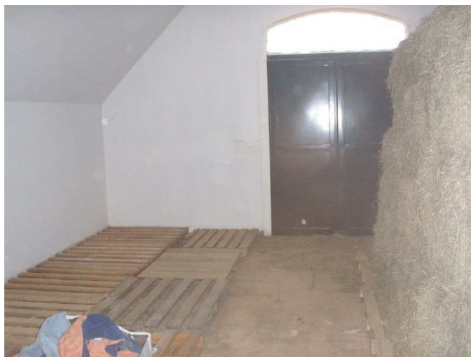
Hay Storage Area (Second Floor)
